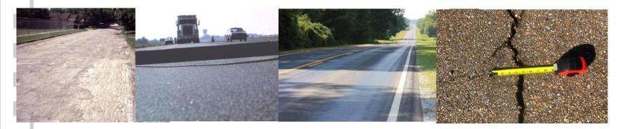
Severely fatigued pavement needs rehabilitation, not a chip seal
